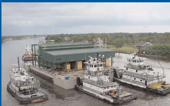
Towing out concrete hull gas module
