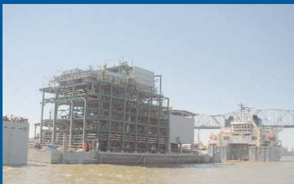
Loading a gas module onto a semi-submersible
